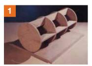
First of all, construct a template out of particleboard. To achieve an exact moulding over the whole surface, keep a maximum distance of 250mm between the ribs.
