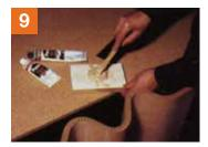
Use a two-component filler to fill the open notches.
